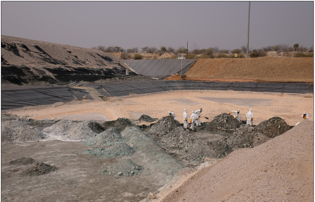
An estimated 300,000 tonnes of toxic waster are stored in Tsumeb. Source Author
