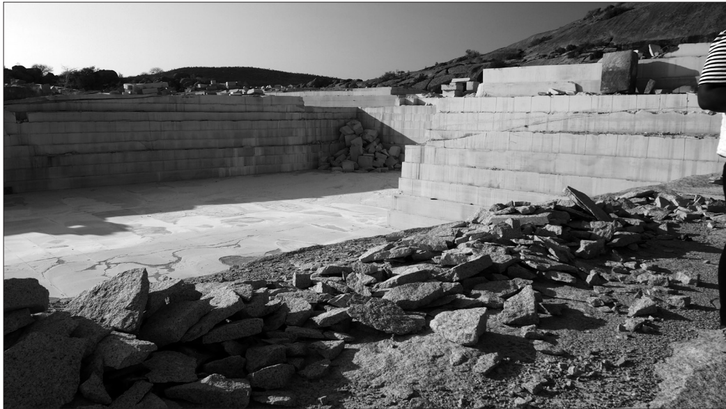
The large pit constructed for rehabilitation was left unused by the mining company.
